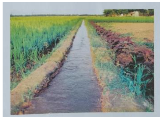
Figure 5: Finished improve earthen canal
