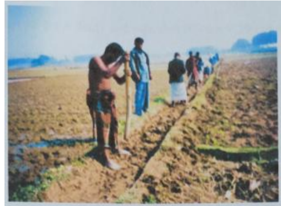
Figure 4: Preparation of improve earthen canal
