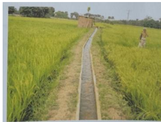
Figure 7: Finished pre-cast rectangular canal
