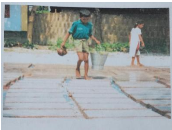
Figure 6: Curing of pre-cast rectangular slab
