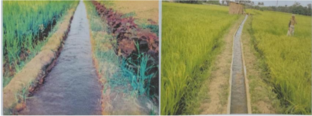
Figure 1: Improved earthen canal (left) and Pre-cast rectangular canal (right)
